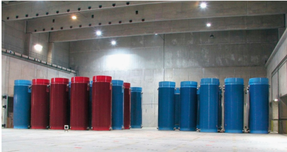
Figure 4-7. Castor container for dry interim storage in a storage building at Gorleben in Germany. The container also fulfils the requirement of being transportable.
