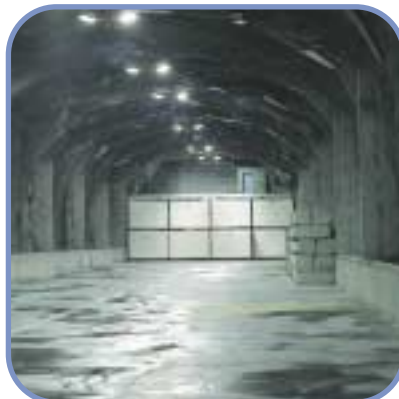
Concrete moulds with intermediate-level waste SFR.
