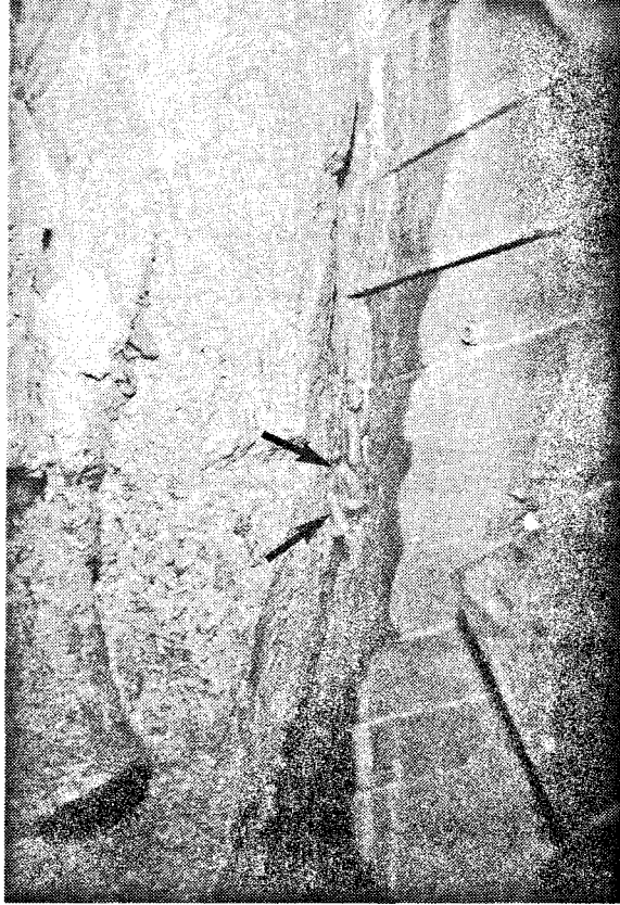
Fig 62. Clay is being pressed out through a fracture (arrow)
